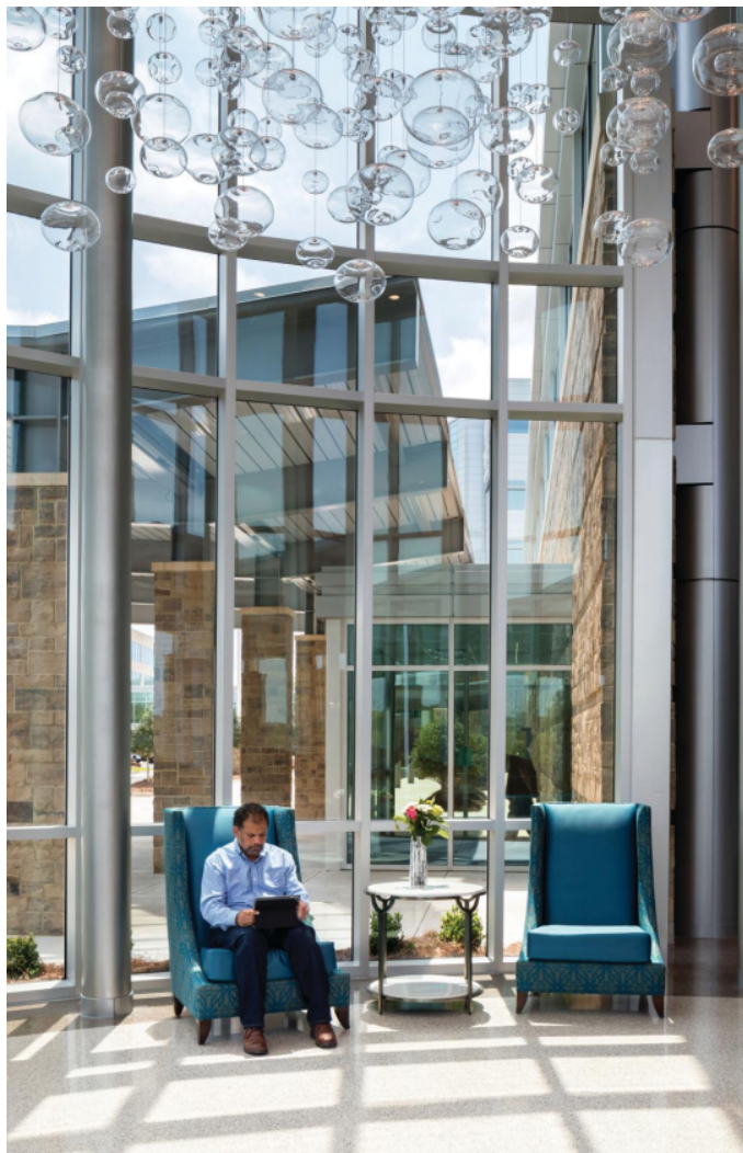
Designed by HDR, Northside Hospital Cherokee in Canton, Ga., automatically adapts to the amount of light with glass that darkens in direct sunlight and increases transparency as daylight reduces.
